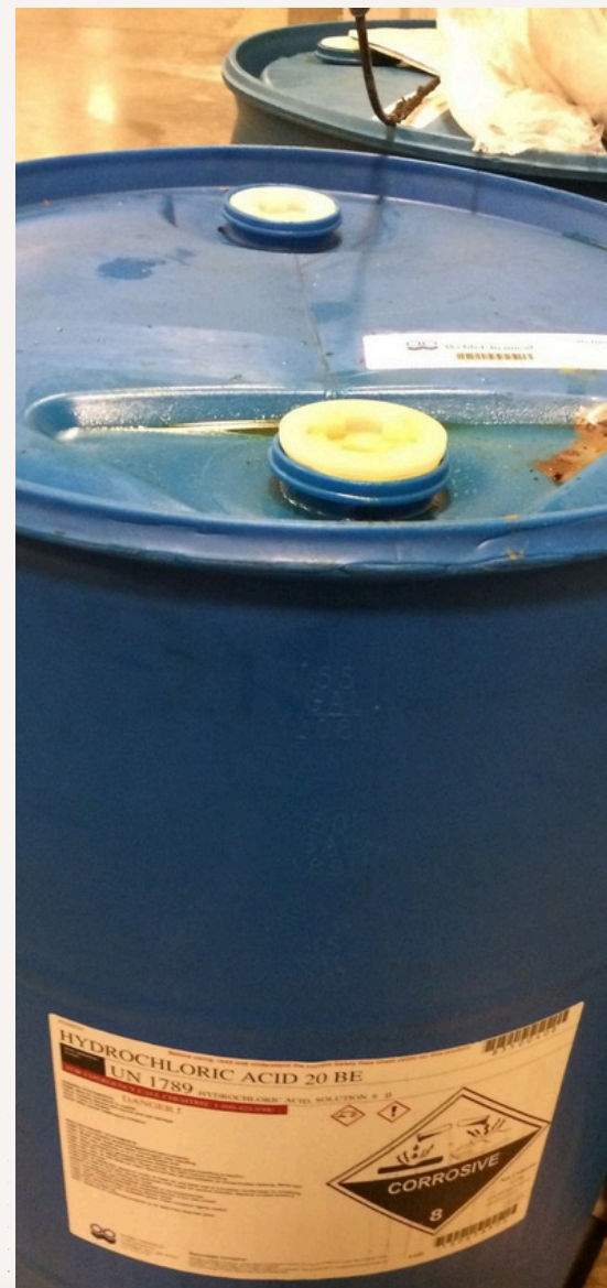
Improper hydrochloric acid (HCl) storage with puddle of acid leaking near the barrel opening at the AquaBounty fish farm in Indiana. Staff were not properly trained in safety procedures. Photo: Braydon Humphrey, April 2019.
